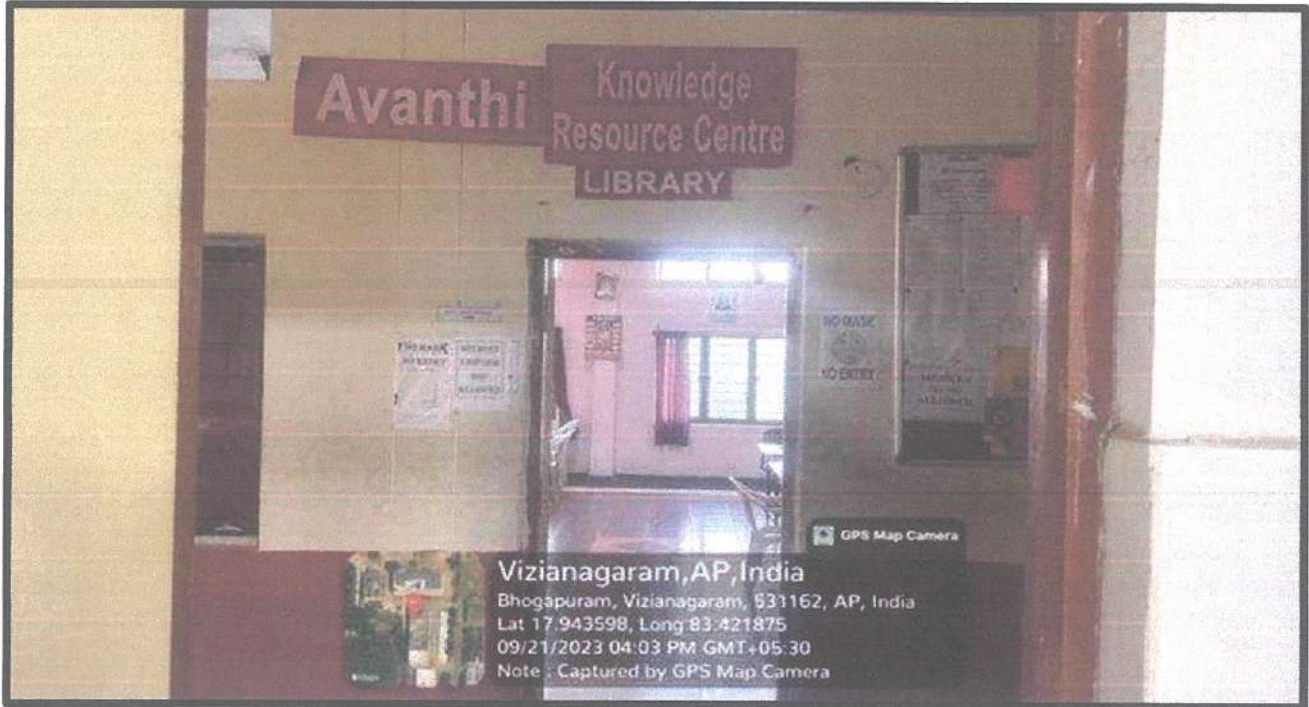
AVANTHI LIBRARY MAIN ENTRANCE
